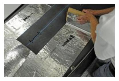
**31.** The sheets were then laid down along these guide lines. This will produce a very straight and neat installation.
