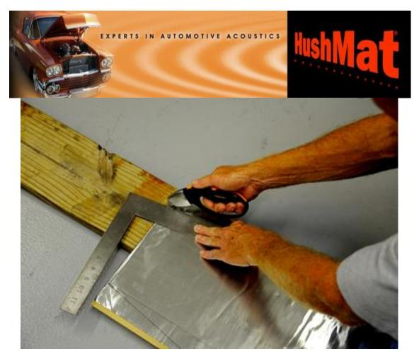
7. The HushMat Ultra can be cut to fit any area using a straight edge and utility knife on a piece of wood as shown here.
