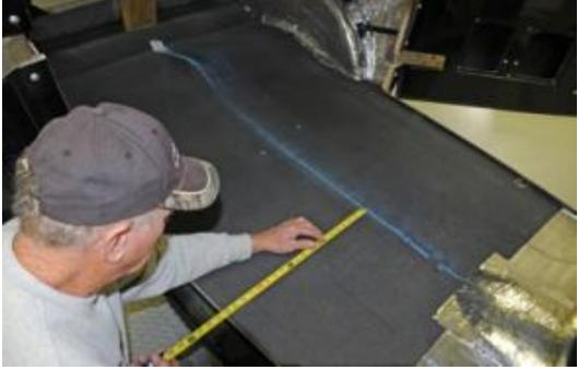
29. Now measure from the center line to determine where the sheets will go to make the best use of all the material and have a neat looking installation.
