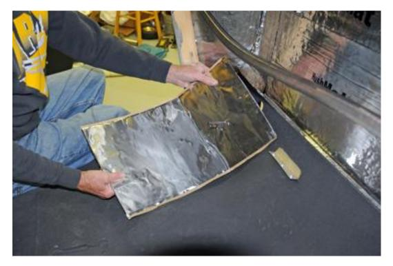
26. The floor is next. The brake pedal arm comes through the floor as most street rods do, so I simply measured where I needed to cut out for it and then slipped the sheet over the pedal arm as shown.
